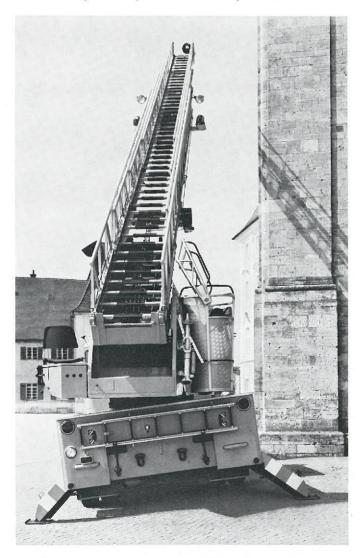
permitting the ladder to also be employed at lower points. The **new levelling feature.** Gimbal-mounted gearing provides perfect ladder set levelling at any elevation between  $-15^{\circ}$  and  $+75^{\circ}$ .
