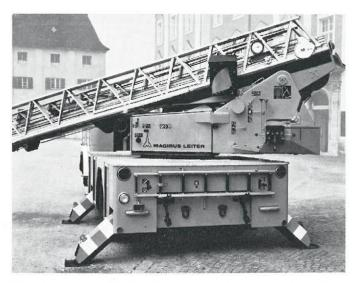
Troublefree control of all ladder movements from a central operating station. Clearly arranged instruments and control levers. Secure stance thanks to the hydraulic inclined stabilizing jacks. The turntable allows the ladder set to be depressed to  $-15^{\circ}$ ,
